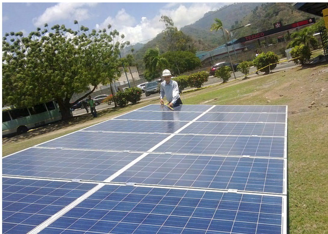
Solar panel installed on the front field, UTech’s Papine campus.
